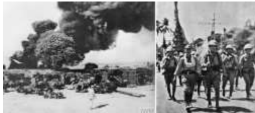
Electrical equipment and oil installations at Yenanguang being destroyed (left) as part of the "scorched earth" policy, in the face of the Japanese advance (right).
